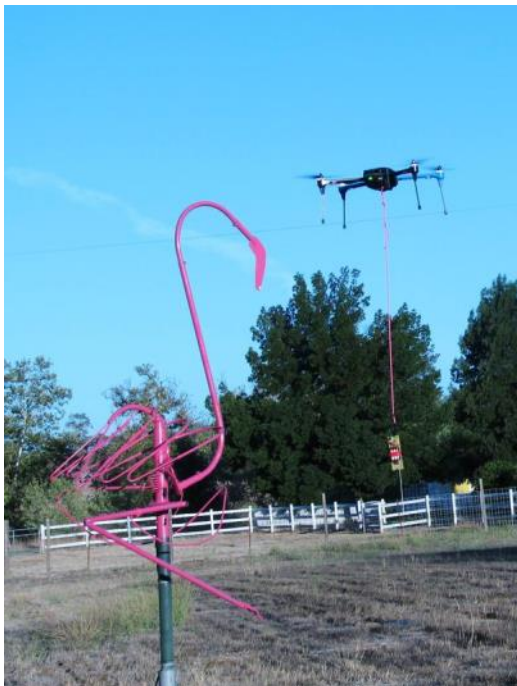
Tom Schiller, N6BT and owner of Next Generation Antennas installing my multi band yagi antenna - 11 elements covering 6 bands (20-10) and 6 meters off the front, as well as a 40 meter rotatable dipole 5 ft above the yagi. The 40 meter does not interact with the antenna below. All is sitting on a 55 ft. tower.
