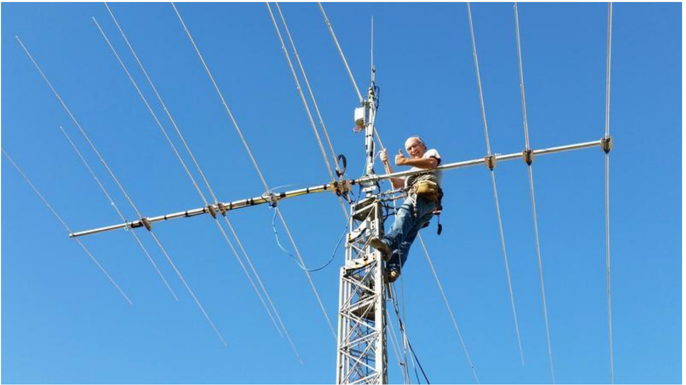
Tom Schiller, N6BT and owner of Next Generation Antennas installing my multi band yagi antenna - 11 elements covering 6 bands (20-10) and 6 meters off the front, as well as a 40 meter rotatable dipole 5 ft above the yagi. The 40 meter does not interact with the antenna below. All is sitting on a 55 ft. tower.
