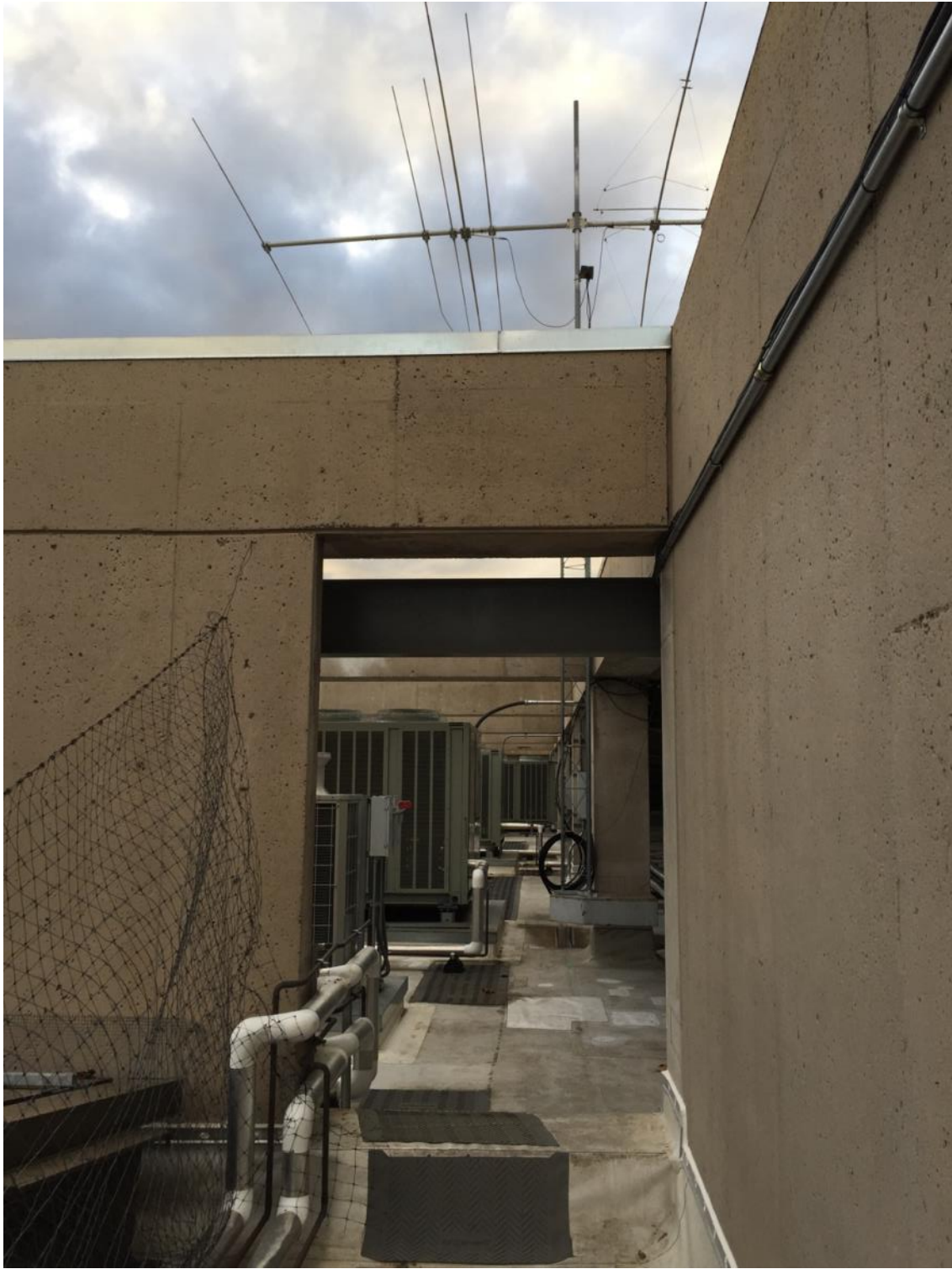
The roof of Hilltop A before removing the existing Yagi – not flat!
