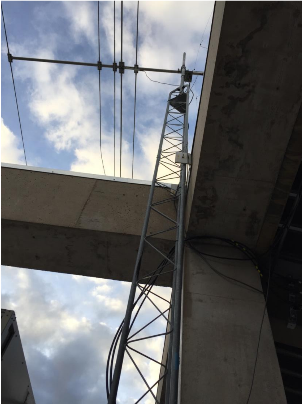
Tower bracketing, with old Force-12 antenna in place
