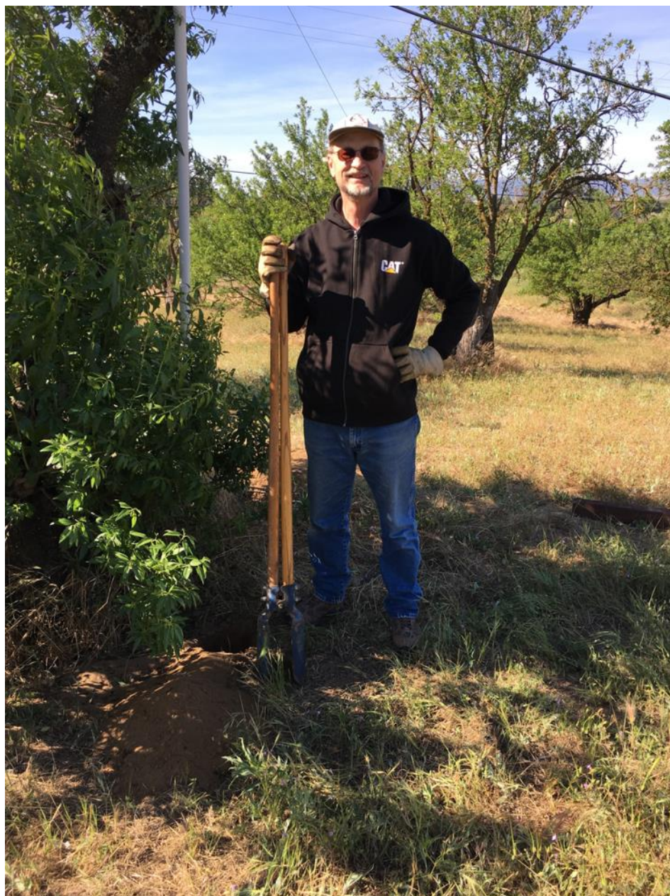
Figure 5. One corner needed its position adjusted, and a new 4x4 support. Here, Gary earns his PhD (Post Hole Digger).
