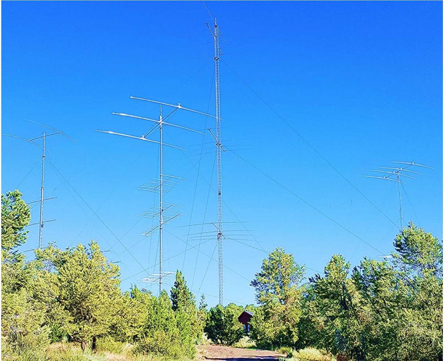
ANT FARM 2018 – Most of the antenna farm seen from the driveway
