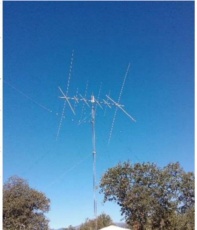
The K6MR Multi-band Quad rests confidently at the top of Ken's 80 foot tower shortly before the 2013 CQP Competition.
